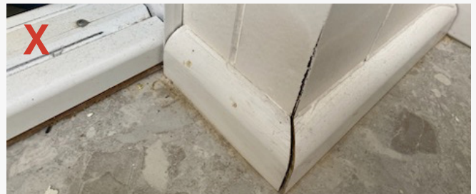
Panel used in a bathroom not installed on top of the skirting resulting in water wicking up the bottom of the panel and damaging it.
