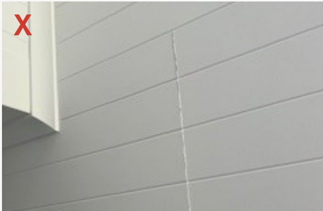
Panel joins showing when panels are installed end to end with no expansion gap or decorative trim cover
